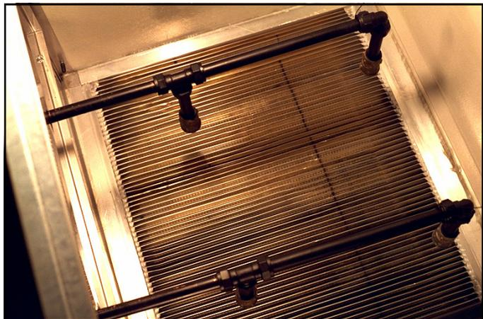
Dependent on the return air wet bulb condition, up to 10 C reduction in supply air can be achieved .
